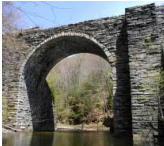
Keystone Arch Bridge © Steve & Linda Hamlin
